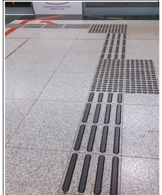
A guidance TWSI consisting of elongated bars arranged in a linear pattern to guide those who are visually impaired to important amenities within a building.
