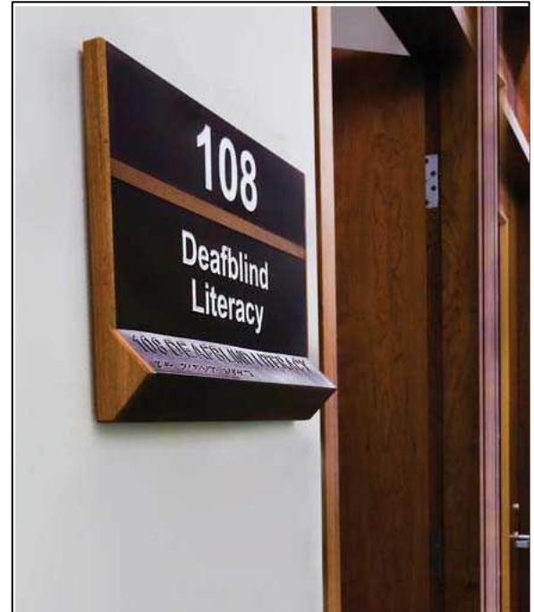
A good example of a sign beside a doorway. The sign provides the same information in print (uppercase and lowercase letters with good contrast to the background), braille and raised print.
